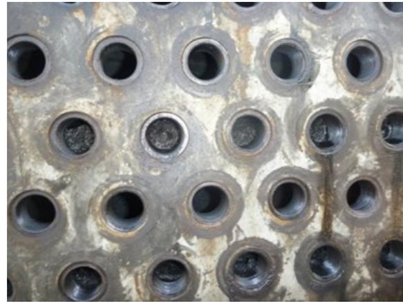
Picture 1: Fouling of cooler tubes
