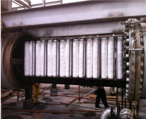
Picture 3: Retrofitted pre-coat filter to cartridges
